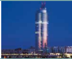
Millennium Tower. AUSTRIA
